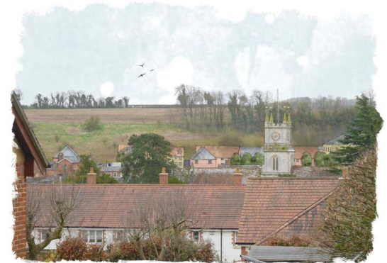
View from across Tabury with the proposed development and embankment in the distance.
