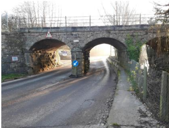
Existing bridge viewed from the Northern side
